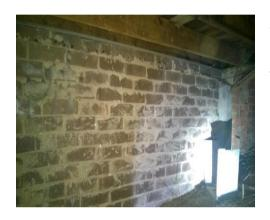
Ant caps are compromised by the enclosed walls in the subfloor. The purpose of ant capping is to reduce the risk of concealed termite attack. The enclosed wall need to be removed and ant capping should be repaired or installed where possible.
