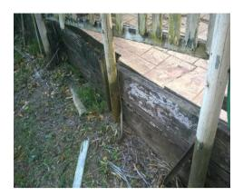
Visible evidence of subterranean termite workings and/or damage was found at the time of inspection. It was in, but not necessarily limited to the following location(s) timber retaining walls at the rear of the garden
