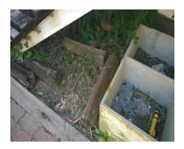
Timbers in contact with the ground, these are susceptible to termite activity. We would recommend removing away from the property
