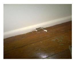
Visible evidence of subterranean termite workings and/or damage was found at the time of inspection. It was in, but not necessarily limited to the following location(s) skirting boards in the lounge
