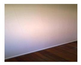
The wall paneling in the dining room is bowing. We would recommend removing the paneling and carrying out a more invasive inspection to determine the course of the problem.
