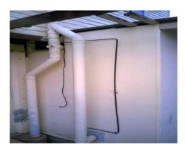
The roofed toilet at the rear has been constructed with no consideration to BCA requirements. We would recommend replacing the enclosure with a structure that complies with current building codes.
