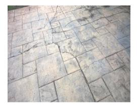
There is cracking & subsidence evident to the concrete patio at the rear of the property, replacement of the concrete is required, consult a concreter for advice
