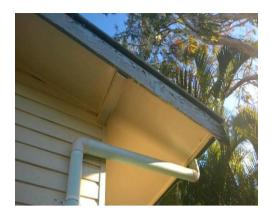
Fascia boards, eaves and barge ends are in poor condition and require repairs and painting
