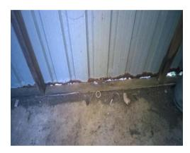
There is corrosion evident to the pool pump housing sheeting, repairs or replacement of the damage sheets is required
