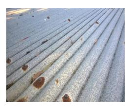
There is surface rusting evident to areas of the roofing sheeting, maintenance will prolong the life of the sheeting but expert advice from a roofing contractor must be sought
