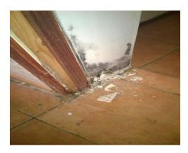
There is mould and plaster damage evident to a door reveal in the garage area. This could be due to water ingress from the roofed area adjacent to this area. We would recommend consulting a roofer for advice
