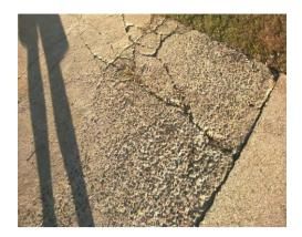
Movement cracks were visible to the concrete driveway, significant repairs are required, consult a concreter for advice
