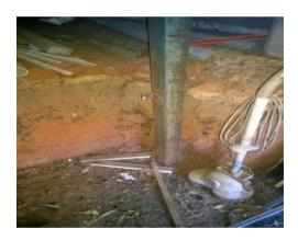
There is rust scale to the steel posts at ground level, Maintenance is required.
