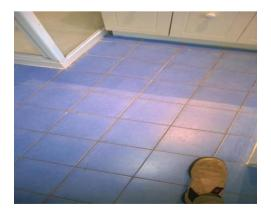
There is cracking to the bathroom floor tiles, maintenance and repair to rectify is required
