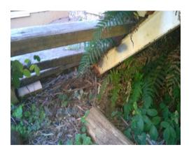
Rusting is evident to the rear staircase stringers & tread brackets, repairs are required. The above recommendation should be implemented as a matter of urgency. Immediate action must be taken to ensure that anyone entering the area is warned of this hazard.
