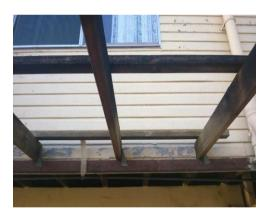
Paint stress is evident to the timber cladding, maintenance is required
