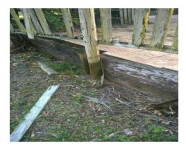
The timber retaining walls at the rear of the garden is out of vertical alignment, replacement of the retaining wall is required.
