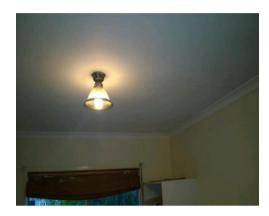
The ceiling lining in the kitchen has been patched. However, further remedial action is required to return the ceiling to a condition commensurate with the other ceilings in the dwelling
