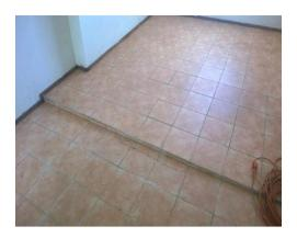
The concrete slab in the enclosed subfloor area is out of horizontal level and has extensive cracking evident to the floor tiles. This could be due to poor site preparation & settlement. We would strongly recommend consulting a licensed builder for advice
