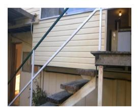
The opening to the Balustrades on the rear staircase have openings greater than 125mm. Openings in the balustrades must be constructed so that any opening does not permit a 125mm sphere to pass through it. This space is tested above the nosing line only, Ref; BCA Part 3.9.2.3 – Balustrades or other barrier construction. The above recommendation should be implemented as a matter of urgency. Immediate action must be taken to ensure that anyone entering the area is warned of this hazard.
