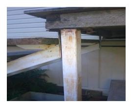
Rusting has caused structural damage to the steel posts on the rear staircase landing and repairs are essential – see a builder for expert advice  $\,$
